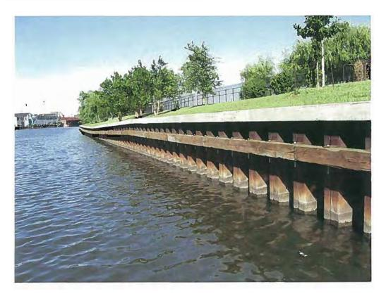
Figure 2-5: Vertical Wall Banks are found throughout the CAWS (photo taken in South Branch Chicago River, near AWQM 40, 2008).
