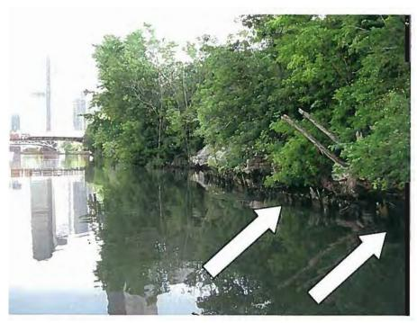
Figure 2-11: Bank Pocket Areas (indicated by white arrows) Created by a Decaying Wooden Seawall on the South Branch Chicago River (photo taken downstream of AWQM 39, 2008).
